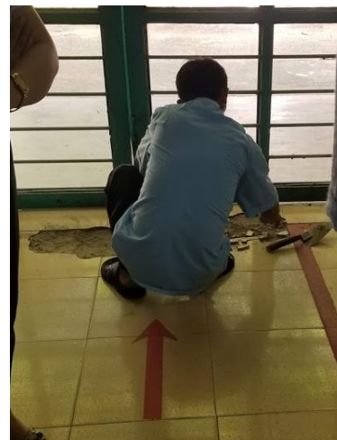
Figure 6: Employee Repairing Broken Flooring
