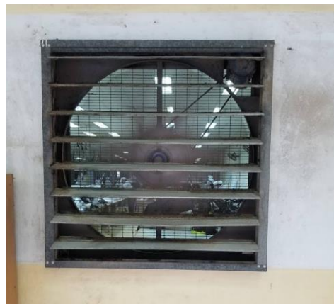
Figure 16: Unguarded Fan Blades inside Dampers
