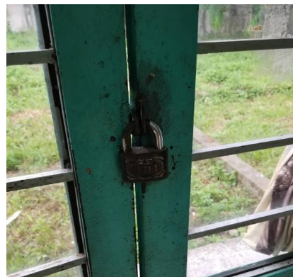
Figure 2: Locked Exit Door
