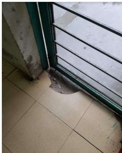
Figures 4 – 5: Broken Flooring at Exit Doorway
