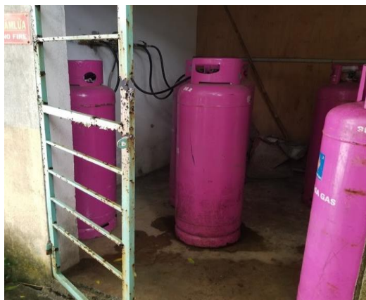
Figure 9: Unsecured Gas Cylinders
