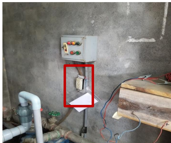
Figures 29 and 30: Ungrounded Electrical Outlet in Fire Pump Room
