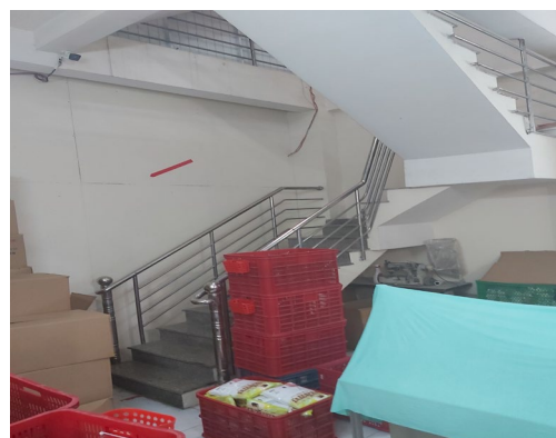
Figure 7: Open stairwell with landing obstructed by flammable boxes and obstructed exit route
