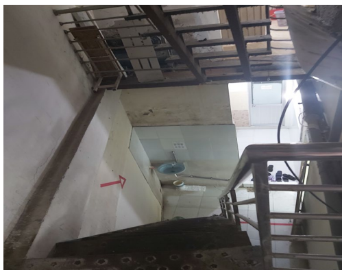
Figure 3: Stairwell exiting to toilet, not building exterior
