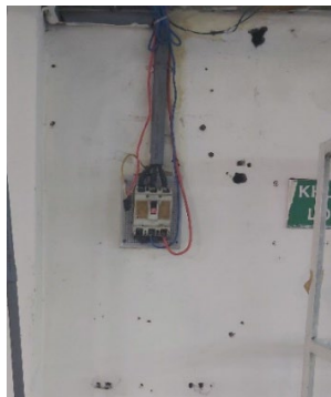
Figure 15: Uncovered electrical switch and wiring
