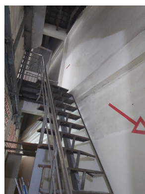
Figure 13: Lack of emergency lighting in stairwell
