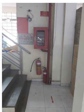
Figures 11 and 12: Fire extinguishers not checked regularly
