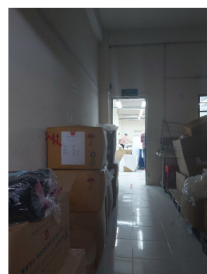
Figure 14: Lack of emergency lighting at and along exit door
