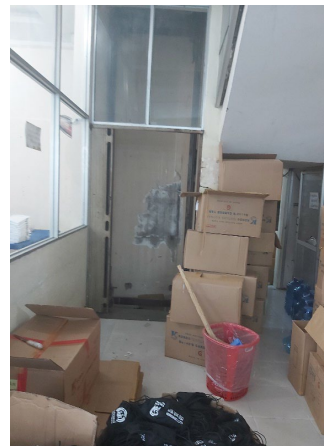
Figure 20: Elevator safety door not closed exposing elevator shaft
