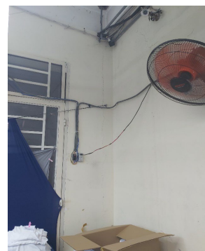
Figures 17 and 18: Uncovered wiring
