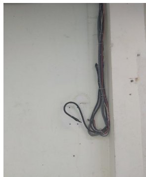
Figures 17 and 18: Uncovered wiring
