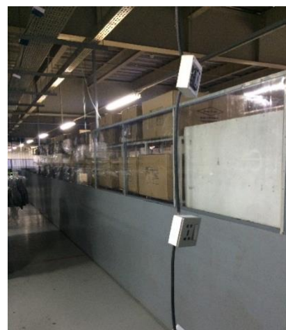
Figure 10: Hanging Electrical Power Sockets at Honeys 2
