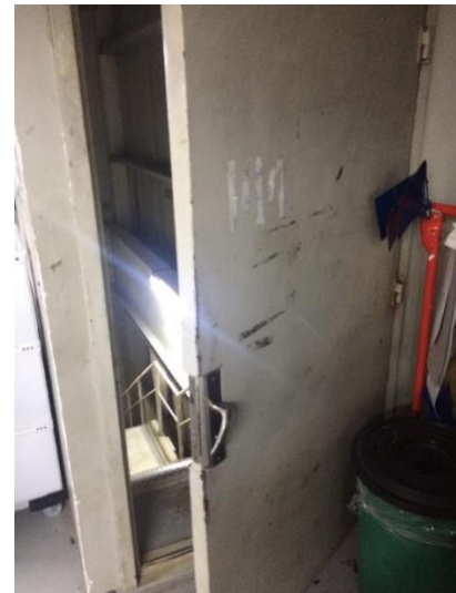
Figure 4: Honeys 2 fire exit door opening inwards
