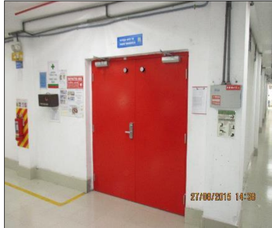
After: Fire door installed
