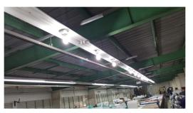
fluorescent tube lights used in this area and throughout the factory. The new bulbs are brighter than the fluorescent lights that were being used and serve to reduce risk of injury to workers in the cutting department by providing increased illumination.
