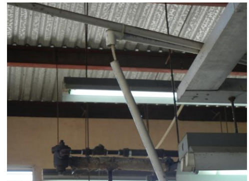
Exposed wires in PVC conduit elbow.
