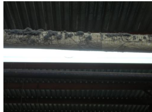
Fabric dust buildup on overhead steam line.
