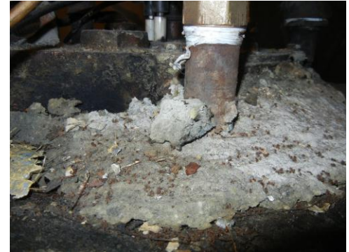
Potential asbestos-containing thermal system insulation on boiler.
