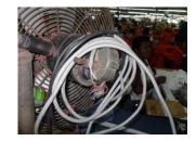
• A second pedestal fan in Building One also is connected by an ungrounded cord. The splice here is also not protected with outer insulation that matches the original cord. Again, there is an accumulation of combustible cloth fiber on the grill of the fan.
