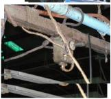
• In Building Two there is fluorescent lighting that has a broken conduit which exposes conductors. The cords to this lighting are hanging low which creates the risk of these cords being snagged.
